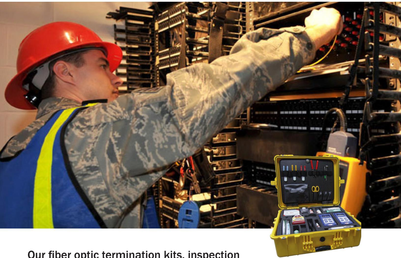
Our fiber optic termination kits, inspection tools, and cleaning supplies allow both lab and field technicians to complete reliable assembly of fiber optic systems. Our termination kits, for example, are equipped with all of the necessary tools—pin and socket polishing tools, jacket strippers, shears, scribes—literally every device required for ongoing termination and test of fiber optic systems. The same holds true for our test probe, inspection and cleaning tools.
