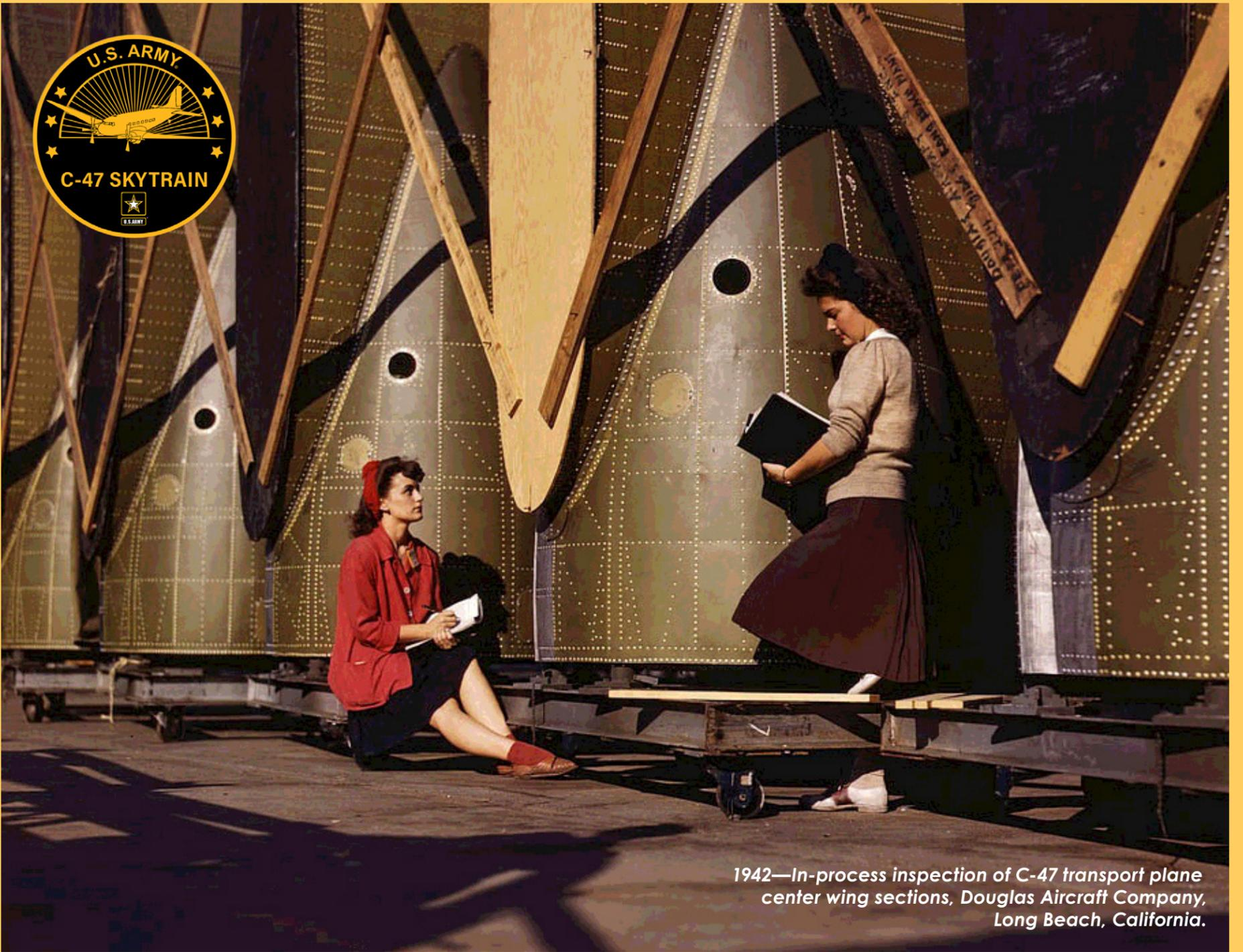
1942—In-process inspection of C-47 transport plane center wing sections, Douglas Aircraft Company, Long Beach, California.
