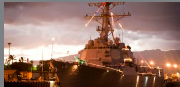
Pier side fiber optic umbilical cable assemblies
